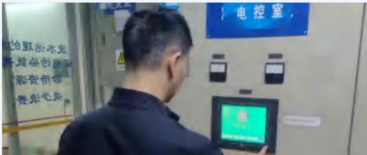
Special emergency drill for excessive wastewater discharge incident at Gree
